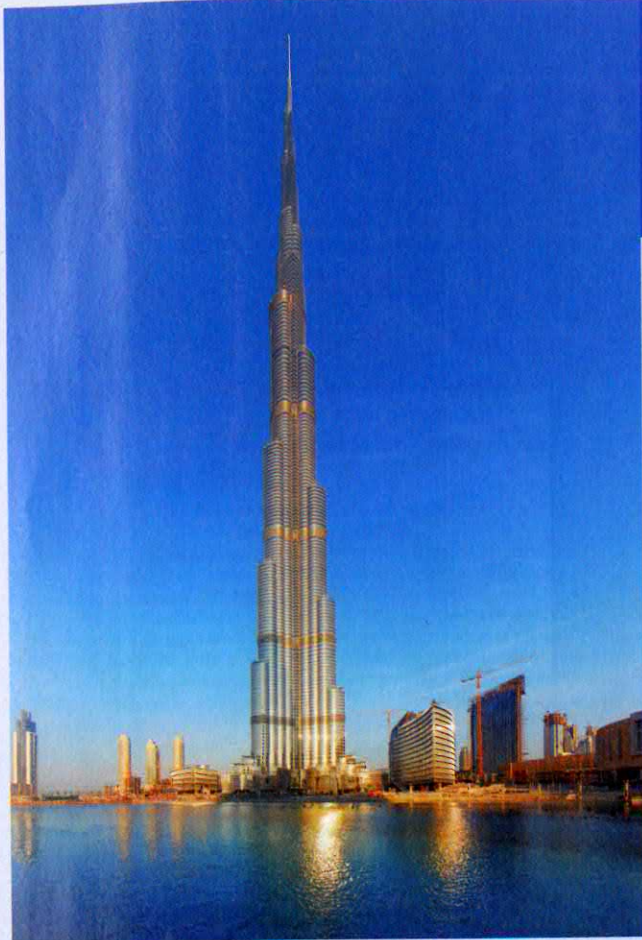
Figure 2. The Burj Khalifa in Dubai, United Arab Emirates (UAE), is, at 828 m, the tallest building in the world. Opened in January 2010, it took more than five years to build. The design includes a variation of cross section with height to help ensure that vortices are not shed coherently along the entire height of the structure. Khalifa bin Zayed Al Nahyan, for whom the burj (tower) is named, is the president of the UAE. (Photo by Nicolas Lannuzel.)
