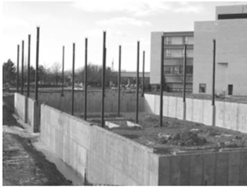
The first structural steel members hoisted were the columns. This is a view of sequence 1 after the columns were set. Notice that all columns have a splice on the top.
