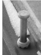
Snow was removed from the locations where shear studs were to be placed (upper left). Using a stud-welding gun (an automatic welding device) the shear studs were then welded to the structural members below the metal decking. Shear studs are used to ensure a composite action between the concrete slab and structural steel beams (upper right). Whether shear studs are used is a function of the structural engineer's design.
