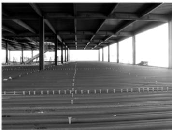
This is a view of the welded studs. Shear studs were tested to ensure that they were correctly welded to the structural steel members in compliance with the bend test of the AWS D 1.1 Structural Welding Code.
