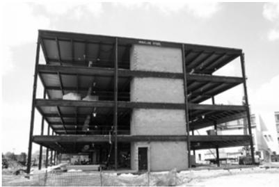
Masonry elevator and stair shafts were installed after the steel frame was erected. The steel frame was secured to the shafts of the building at each floor providing lateral stability for the frame.
