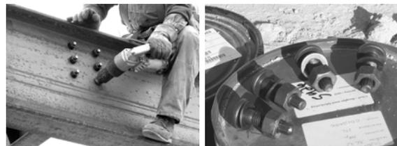
After a section of the structural frame was assembled and vertically aligned, ironworkers permanently fastened the structural steel members with additional bolts and welds. Tension controlled bolts (F1852) were used. Final bolt-up was performed using a torque wrench. The wrench stops automatically when the bolt shears at a tension control groove indicating that the required tension is reached.
