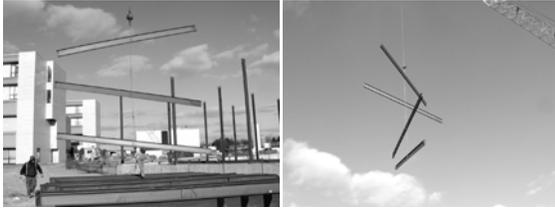
Multiple lift rigging is a process used to hoist several pieces of steel simultaneously. This is accomplished by utilizing a rigging assembly that facilitates the attachment of up to five independent loads to the hoist rigging of a crane. In this project up to four beams were hoisted at a time. Multiple lift rigging speeds the lifting process by reducing the total number of lifts required for the frame.
