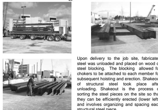
Upon delivery to the job site, fabricated steel was unloaded and placed on wood or steel blocking. The blocking allowed for chokers to be attached to each member for subsequent hoisting and erection. Shakeout of structural steel took place after unloading. Shakeout is the process of sorting the steel pieces on the site so that they can be efficiently erected (lower left), and involves organizing and spacing each structural steel piece.
