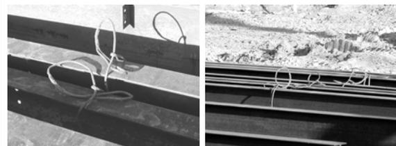
A choker is a rigging assembly used to attach a load to a hoisting device. It is usually made of wire rope or synthetic fiber. Chokers are used to hoist beams into position. They are positioned at the center of gravity of the beam so that the beam remains level when hoisted.
