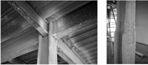
Structural steel has to be protected from fire. Steel will not burn, but it may become soft and weak when exposed to intense heat. Building codes regulate the need for fireproofing and its required locations. There are several methods for fireproofing. The method used for this project utilized spray-on fireproofing. Spray-on material may be portland cement or a gypsum-based product and can be applied directly to structural steel members.
