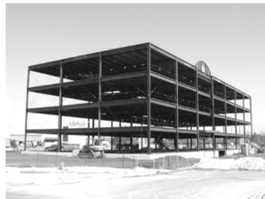
The structural steel frame was inspected upon completion by the local jurisdiction and work could proceed accordingly. Depending on frame complexity, additional periodic inspection and testing may also be required by the local jurisdiction. The design engineer also conducts contract administration and field observation activities which help ensure quality.
