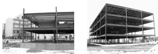
Temporary bracing was placed before plumbing up the structural frame. Temporary bracing is used to provide temporary lateral stability to the structure and to plumb up the frame. The temporary bracing was removed by the erector once the structural steel frame was secured to the vertical masonry elevator and stair shafts, which were installed after completion of the steel frame.
