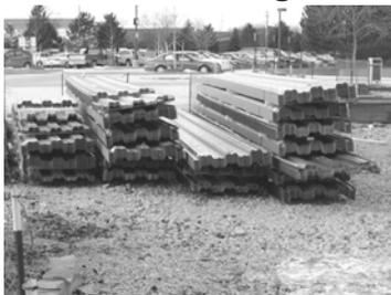
This is the metal decking used in the project. The erector had the responsibility of unloading and hoisting metal decking to pre-established positions on the frame.
