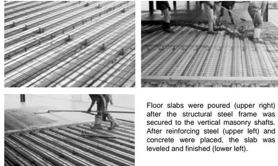
Floor slabs were poured (upper right) after the structural steel frame was secured to the vertical masonry shafts. After reinforcing steel (upper left) and concrete were placed, the slab was leveled and finished (lower left).
