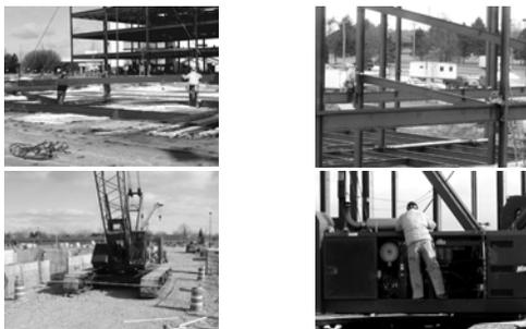
Seven people formed the erection crew used for this project. The crew consisted of one foreman, two ironworkers hooking steel (upper left), two ironworkers connecting steel (upper right), a crane operator (lower left), and an oiler (lower right).
