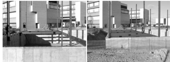
Main girders are hoisted after the columns. Beams are then hoisted and connected to the girders. On the left is a photograph of the first bay to be hoisted. On the right is a photograph of the first three bays in place.
