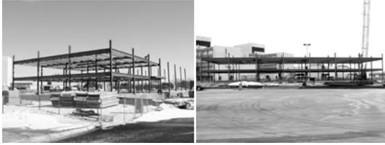
This is a view of the completed hoisting activity for sequences 3 and 4. Hoisting these two sequences took approximately 9 days in contrast with the five days it took to hoist sequences 1 and 2, because sequences 3 and 4 consisted of two floors (365 pieces of steel) and sequences 1 and 2 consisted of one floor (166 pieces of steel).
