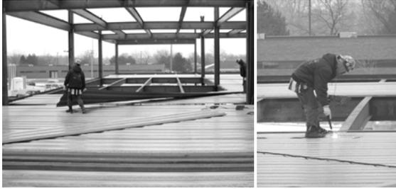
Metal deck was placed and attached with a series of welds. Controlled deck zones were used during installation. A controlled deck zone is an area in which initial installation and placement of metal decking may take place without the use of guardrail systems, personal fall arrest systems, fall restraint systems, or safety net systems and where access to the zone is controlled.
