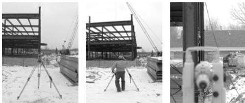
Plumbing up refers to the vertical alignment of the structure. A theodolite was used to verify the alignment of columns in the perimeter of the building. The foreman directed ironworkers on the structure to shift the frame using the temporary bracing.
