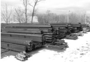
After fabrication, finished structural steel members are stored in the fabricator's storage yard. The more organized the yard, the easier it will be to transport steel to the site. In this case structural steel was stored according to erection sequence. Sequences define areas of the frame and are used to organize their delivery and erection. The practice of planning and storing by sequence improves the efficiency of loading, delivery, offloading and erection.
