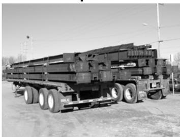
Once the on-site crane was fully set up, the fabricator loaded the steel members for sequence 1 onto trucks and transported them to the job site. Structural steel was delivered by sequence throughout the erection process. It took a total of 29 truckloads to deliver all of the structural steel for the project.
