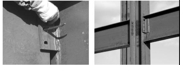
The connector uses pins to align the holes between structural steel members being connected. Then he places several bolts and temporarily tightens them with his spud wrench. At least two bolts per connection are used to temporarily fasten each connection.
