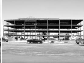
This is a view of the completed hoisting activity for sequences 5 (left) and 6 (right). It took approximately 9 days to hoist both sequences, similar to sequences 3 and 4.
