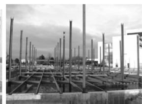
This is a view of the completed hoisting activity for sequences 1 (left) and 2 (right). It took approximately 5 days to hoist the 166 pieces of steel that are part of the two sequences.
