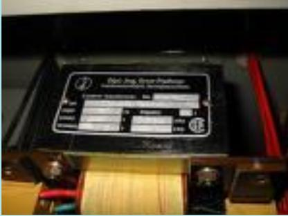
Transformer nameplates contain information about the size of the transformer in terms of how much apparent power (rated in kVA) it is designated to deliver to the load on a continuous basis as well primary and secondary voltages and currents.
