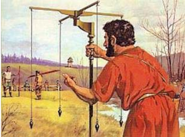
Figure 15 a gorma being use to project a line forward
