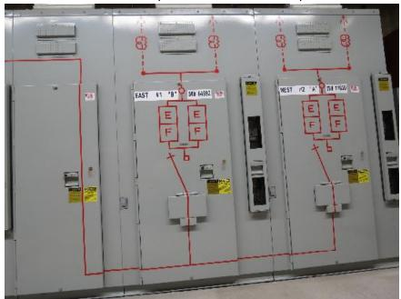
Figure 2: Bay 7 (center) and Bay 8 (right) of the Vault 24 switchgear lineup.
