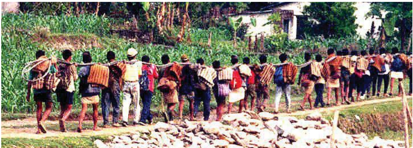
Transporting a cable on the Shoulder (for short distances).
