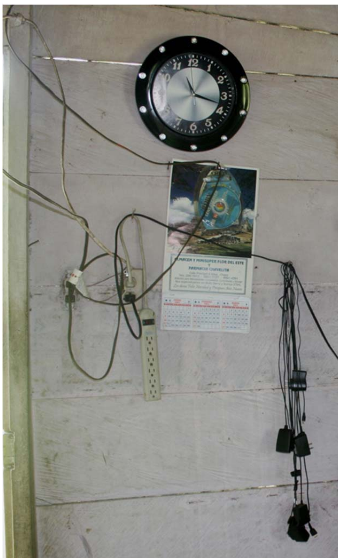
Figure 9: Sample of Current Electrical Wiring Within Homes
