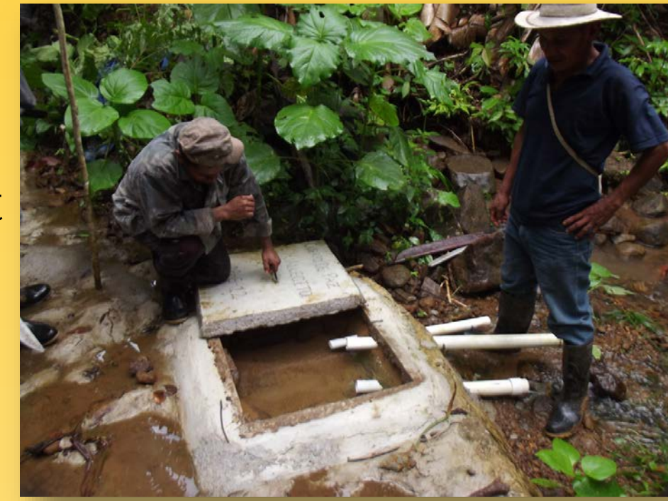
Figure 4: Existing spring box
