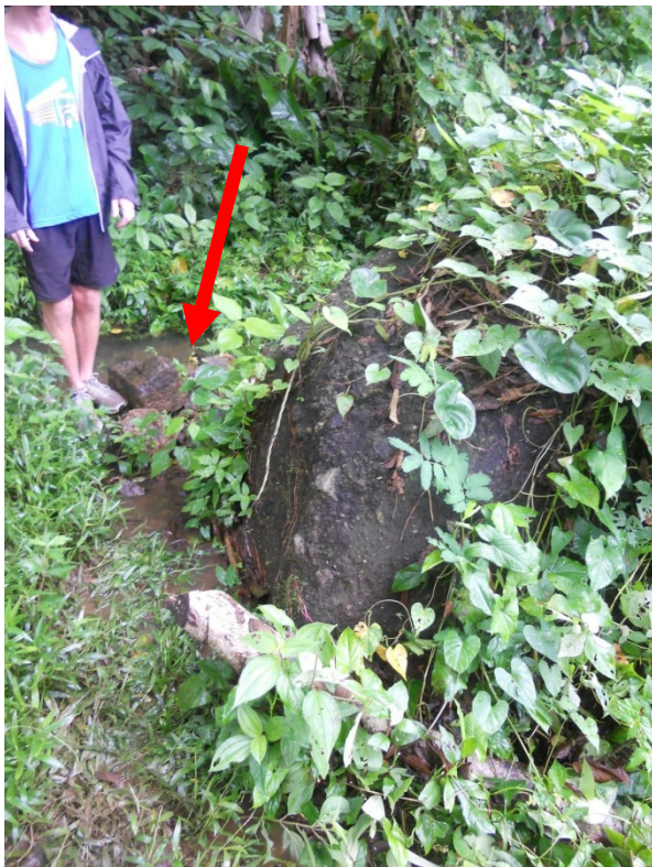
Figure 9. The Quebrada system dam will be constructed in place of the current temporary dam put together by the community members (indicated by red arrow)
