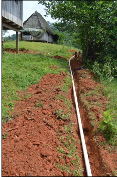
Figure 19. Photograph showing a pipe within a trench at Bajo Gavilan. The trench will be filled to bury and protect the pipe [10].
