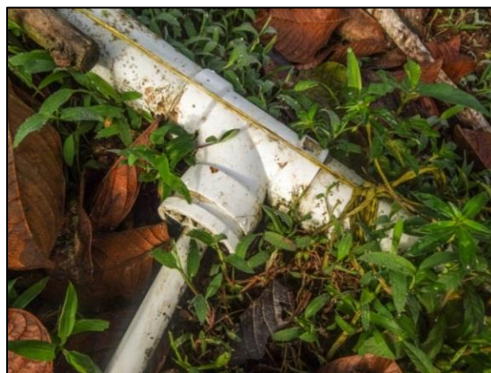
Figure 27. Tee fitting to branch off 1.5" mainline to tapstands.
