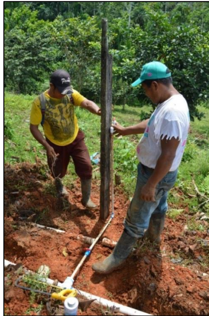
Figure 28. Tapstand built in section 3 of the community [10].
