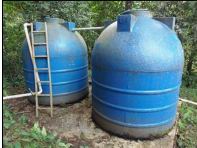
Figure 26. Two 4,200 L storage tanks located at the existing aqueduct.
