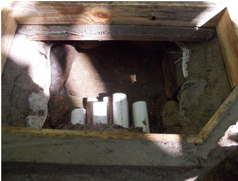
Figure 9: Access hatch space. It's easiest if the access hatch is square or rectangular, but sometimes it ends up being a different shape, which is fine.
