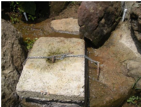
Figure 12: Access hatch lid on raised lip.
