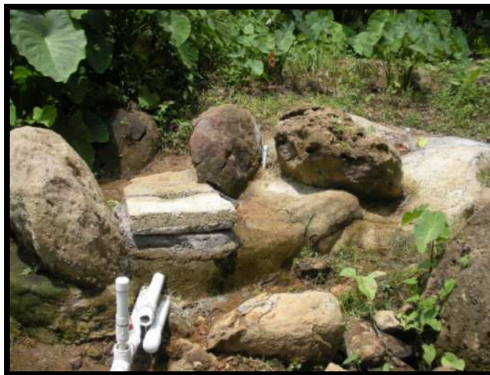
Figure 8: Low-Profile Spring Box from Snyder report in Appendix D.
