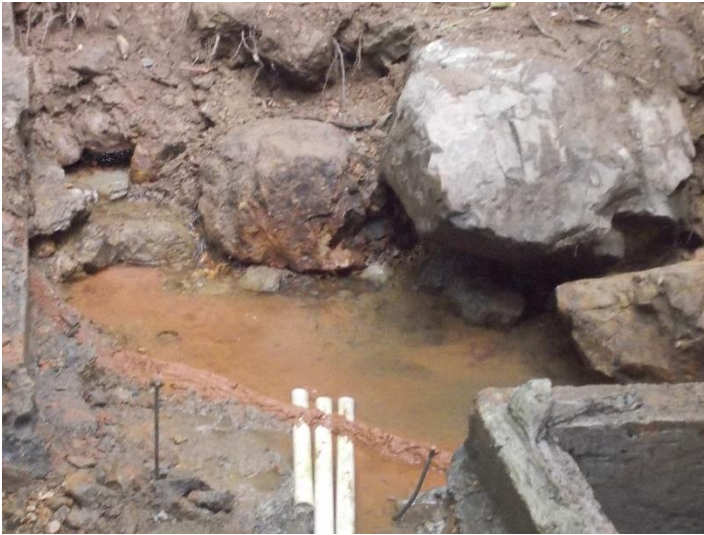
Figure 7: Picture of clay wall with pipes. This clay wall still needs some work because the area just downstream of the clay wall where the actual wall will go still has water.
