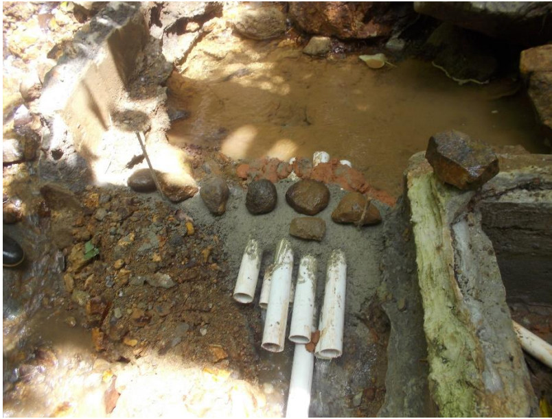
Figure 8: Stone masonry construction for wing walls. (This toma has more exit pipes than normal; just ignore that.)
