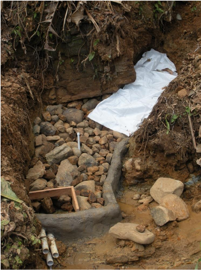
Figure 10: Toma filled with rocks and beginning to be covered with sacos before pouring the concrete slab.
