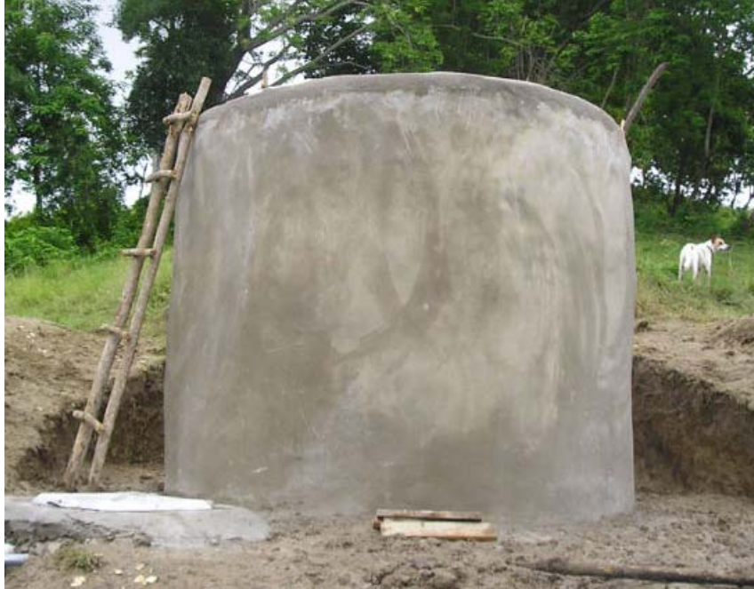
Figure 5: Ferrocement Tank (Water Charity, 2010)
