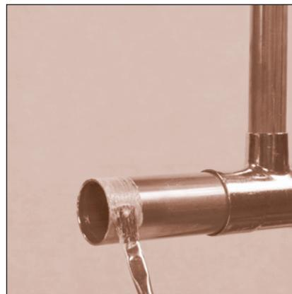
FIGURE 18: Fluxing: Tube
