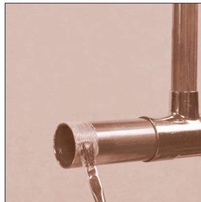
FIGURE 18: Fluxing: Tube
