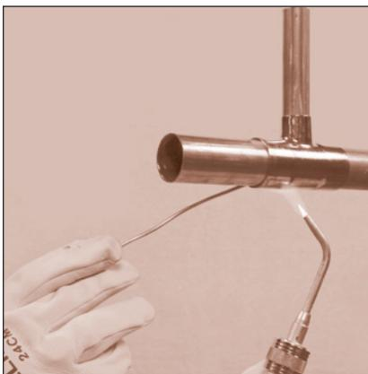
**FIGURE 25: Soldering**
