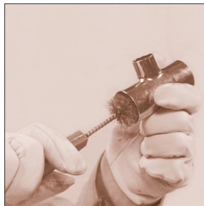
FIGURE 17: Cleaning: Fitting Brush
