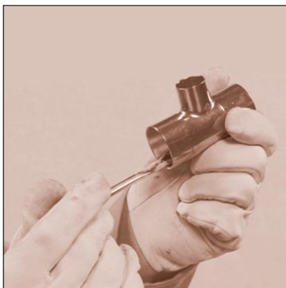
FIGURE 19: Fluxing: Fitting
