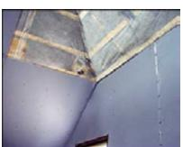
Blueboard's characteristic hue comes from a special plaster-friendly paper applied over its gypsum core.
