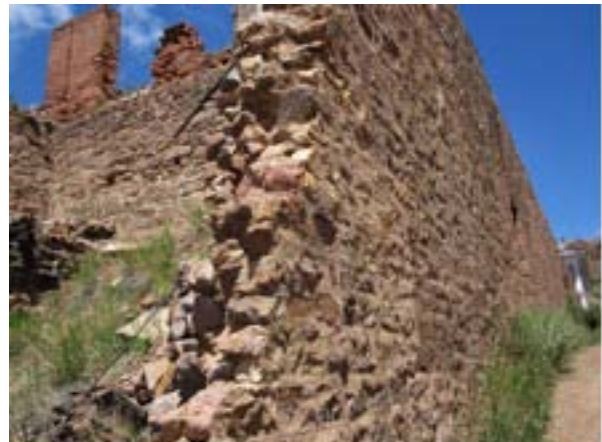
The back of the Gold Coin Mine constructed of local Precambrian granites
