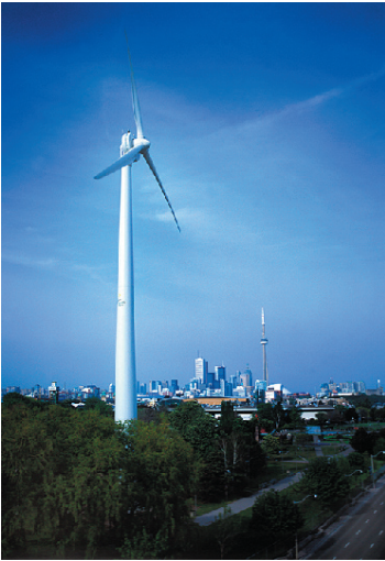
Urban-sited community wind, Toronto's WindShare project. (Photo courtesy Toronto Hydro)
