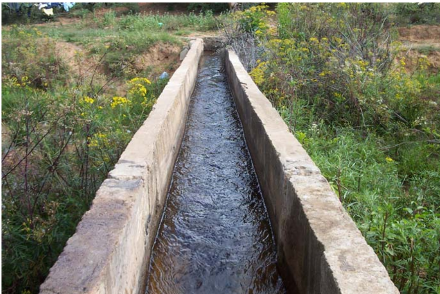
Figure 6.5: As is the case in many Bolivian communities, this irrigation canal is the lifeblood of Tipa Tipa
