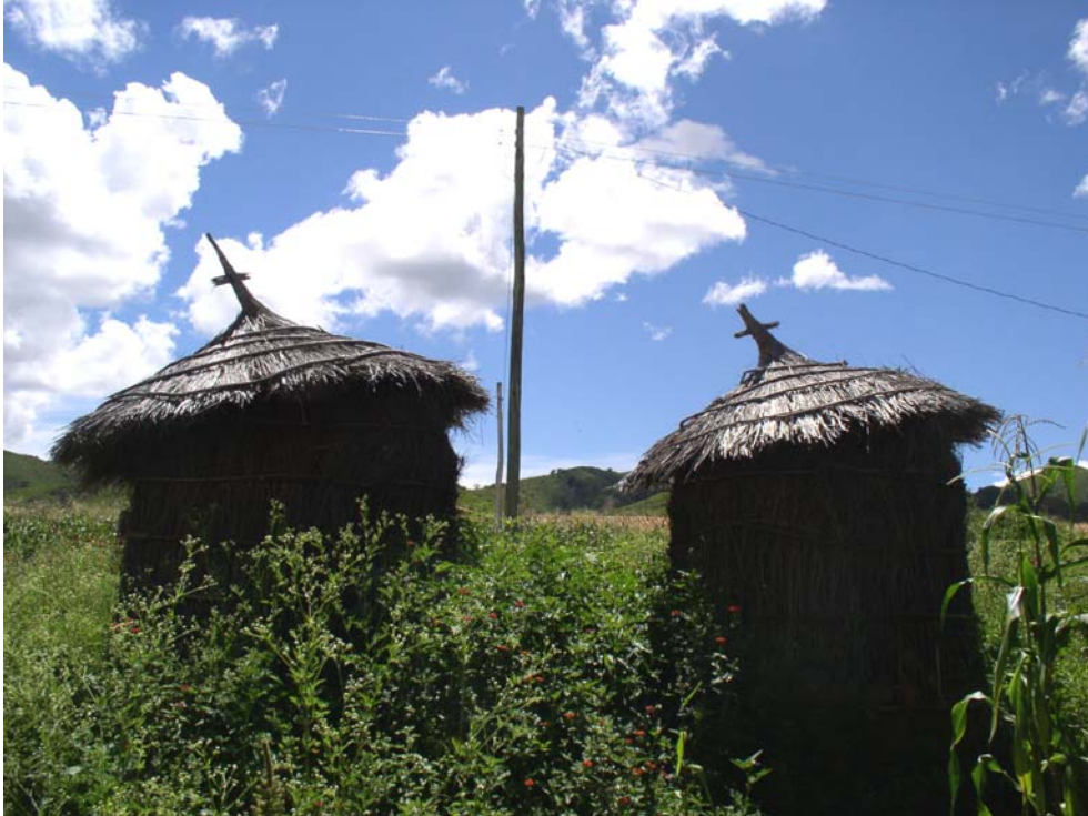
Figure 6.1: Called a pirhua in Quechua, these silos have detachable roofs to allow for easy access to the stored maize
