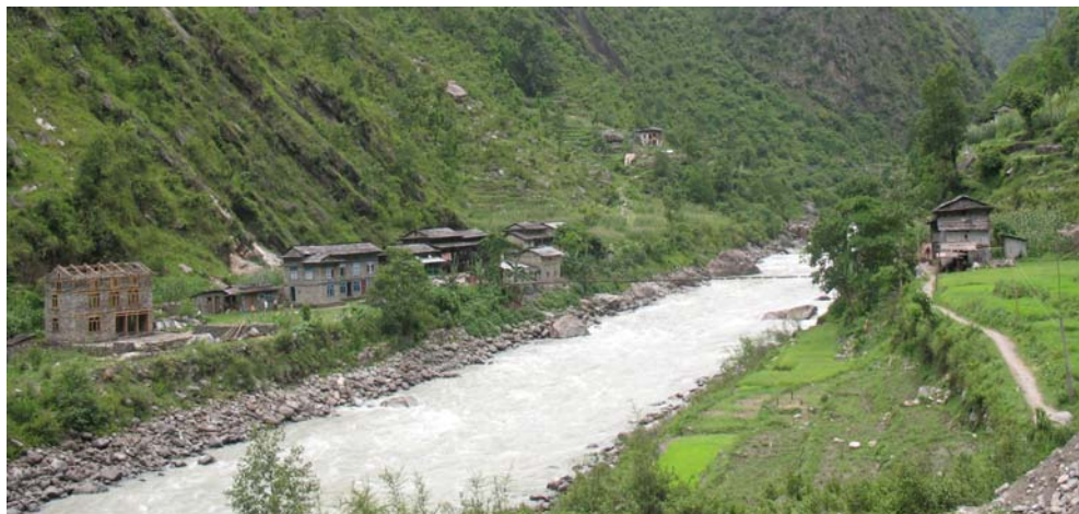
Figure 3-2. Houses, trail, and infrastructures such as the suspension bridge that are in the GLOF hazard zone at Jagat. (Photo by author)
