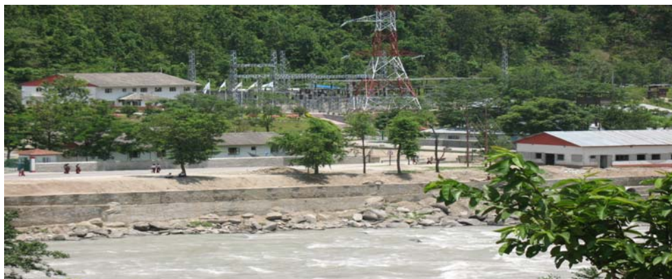
Figure 3-3. Structural mitigation adjustment to protect Khimti Hydro-power plant at Khimti (Photo by author)
