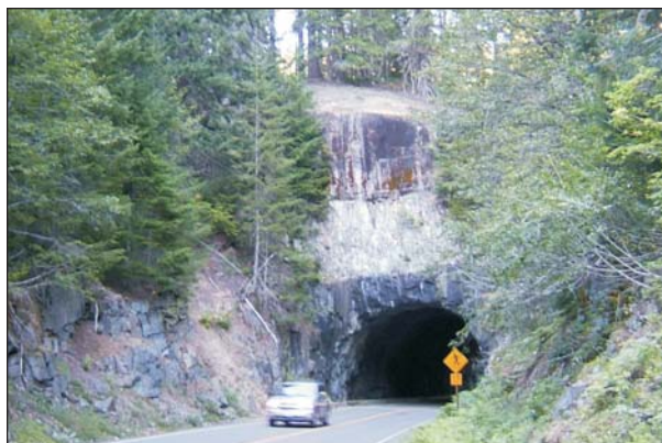
Figure B-12. Dark-colored sill about 10 ft (3 m) thick at the top of the west portal of the highway tunnel west of Box Canyon. According to Fiske and others (1963), here a Tatoosh sill is cutting a Fife's Peak Formation sill.
